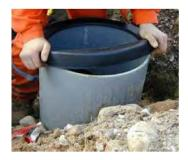
1. Check the chamber throat and remove any debris from the inside or outside of the pipe.
