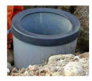
2. Make sure the ring is well seated by pushing down firmly onto the ring all around.
