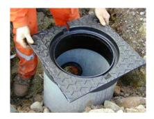
6. Once the correct height is achieved, pour concrete around the cover and chamber as shown in the below diagram.
