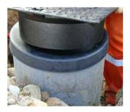
3. Apply a small amount of standard pipe lubricant to the ring surface. Place the inspection cover in the centre of the ring and push down vertically until the inspection cover enters the seal.
