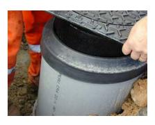
5. Ensure the ring is prevented from dislodging when lifting the cover up for adjustment.
