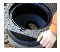
4. Adjust the cover as required by lifting the cover up or pushing down further.
